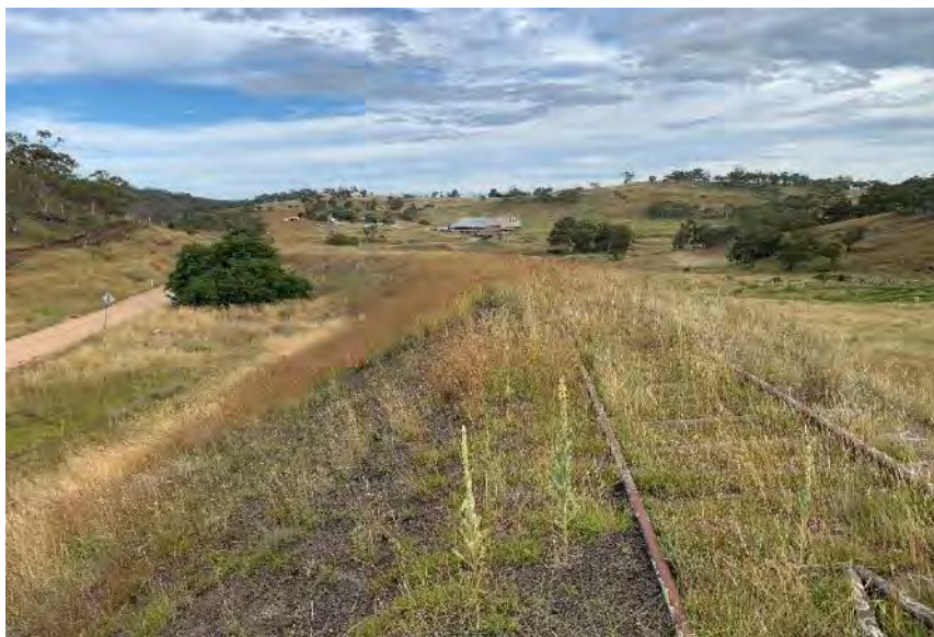
Figure 11-8: View of overgrown approach.
