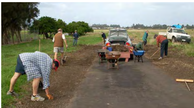
Volunteers organised by the Committee of Management at a busy bee to undertake maintenance work along the rail trail near Port Fairy in Victoria.
