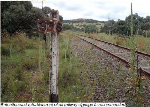
Retention and refurbishment of all railway signage is recommended
