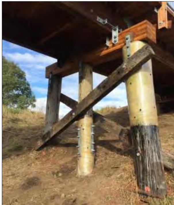
Figure 12-8: Diffuser (Borate Salt) rods are installed in the remaining hardwood elements to resist further deterioration of the timber caused by fungi growth. Note the red bungs are the decay ‘hotspots’ where the timber is prone to have a higher moisture content. These holes are required to be checked for rod depletion as per the issued maintenance manual (typically every 2-5 years depending on environmental conditions).
