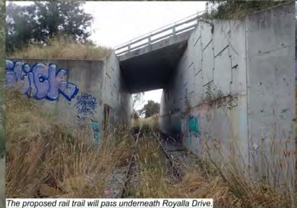
The proposed rail trail will pass underneath Royalla Drive.
