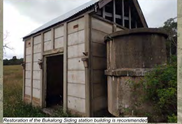
Restoration of the Bukalong Siding station building is recommended
