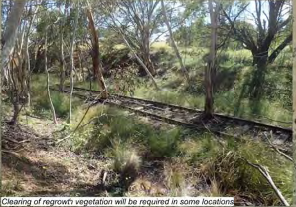
Clearing of regrowth vegetation will be required in some locations
