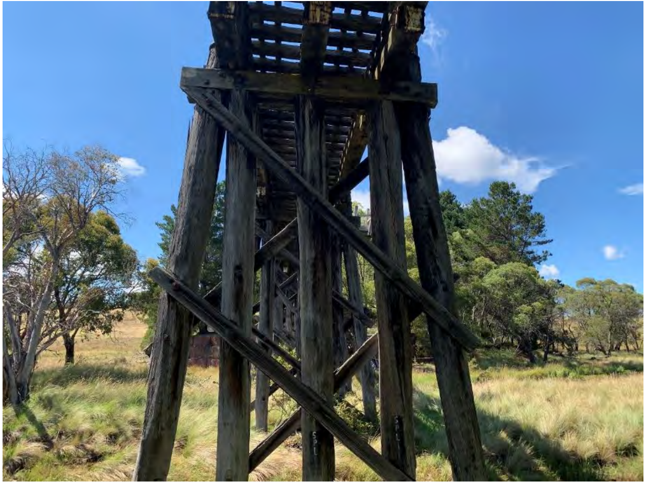
Figure 10-2: View of the timber pile bents configuration. Each pile bent comprises of 5 driven piles (3 Plum piles directly under the girders and 2 batter piles on either side) and are supported by double cross bracing (“X” at top and bottom of piles) and timber wales at the bottom. The two abutments do not contain the cross bracing and only exhibit 3 plum piles. It was noted that significant water stains were present on all timber members of each pile bent. This indicates a high moisture content, when timber elements reach 22%, decay causing fungi are activated and the decay process begins. Overall, the timber bents were found to range from fair to poor condition. Sapwood decay is present at on the piles within the image above. Note that the cross braces do not go all the way to the head stocks.
