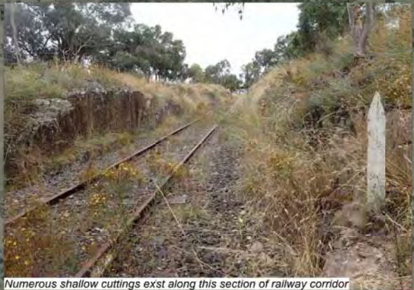
Numerous shallow cuttings exist along this section of railway corridor
