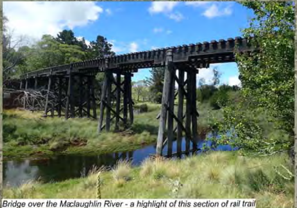
Bridge over the Maclaughlin River - a highlight of this section of rail trail
