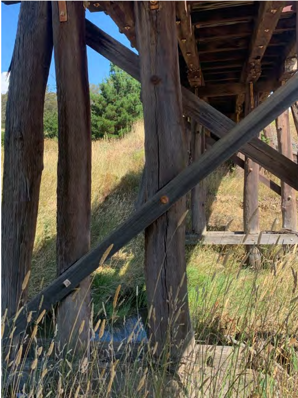
Figure 8-7: View of timber pile and cross bracing connection.
