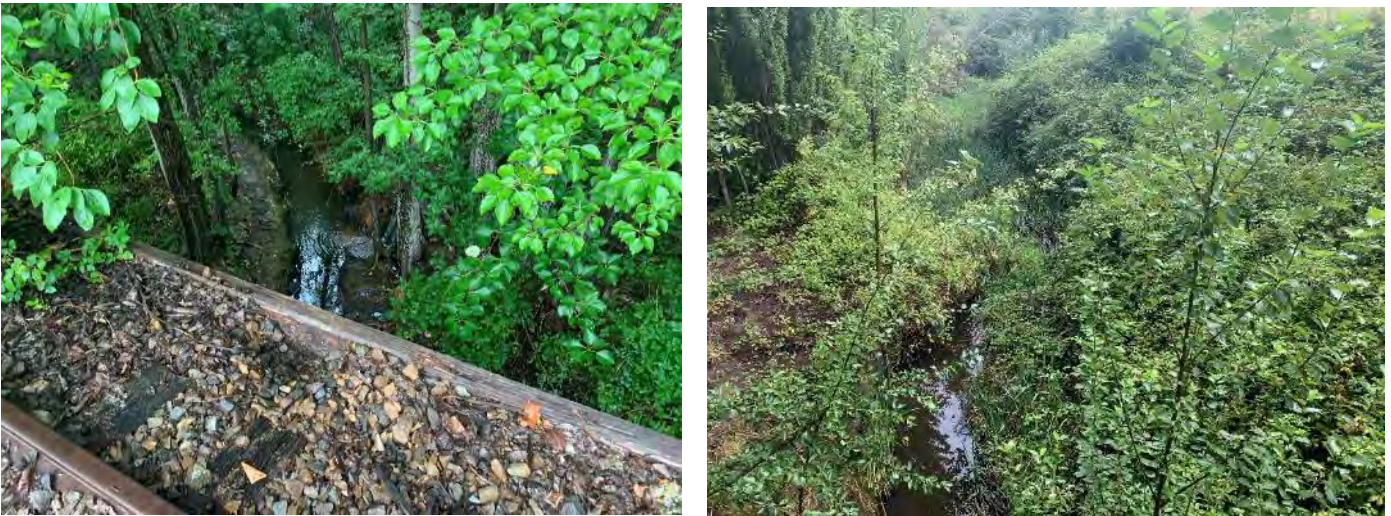
Figure 4-9: Left photo is the general downstream view from bridge deck & photo on the right is the upstream view.
