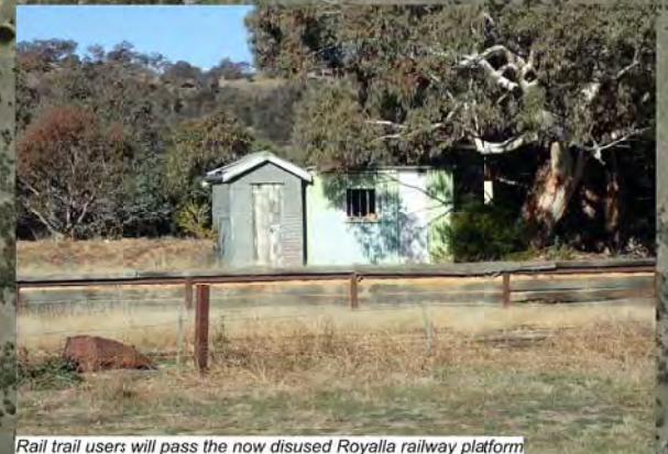
Rail trail users will pass the now disused Royalla railway platform
