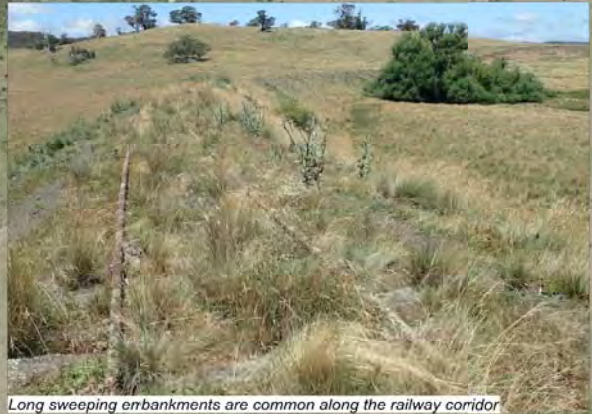
Long sweeping embankments are common along the railway corridor
