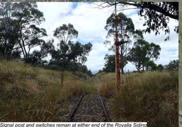
Signal post and switches remain at either end of the Royalla Siding
