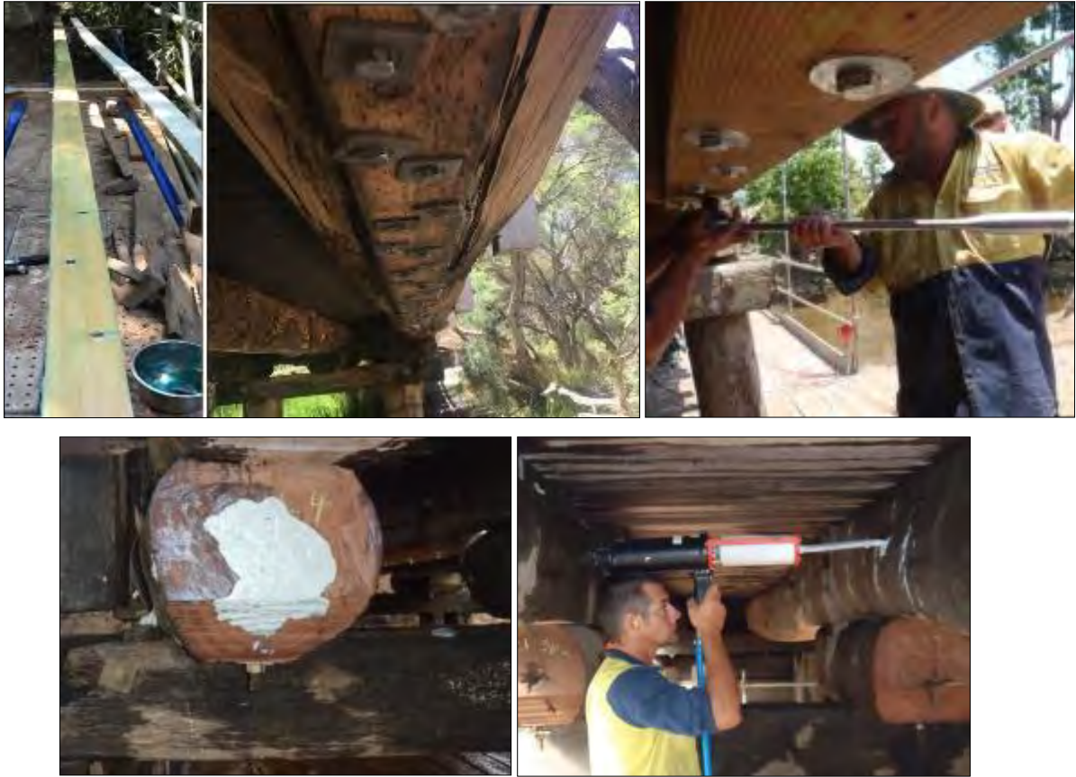
Figure 12-5: The repair of Meachams Bridge in Cassowary Coast. The bridge was retrofitted with fibre reinforcement on the bottom of the girders, some corbels and girders were injected with a high strength epoxy. Some piles were also wrapped with high strength fibre and injected with epoxy, then the entire bridge was diffused with borate salt rods to neutralize decay growth.
