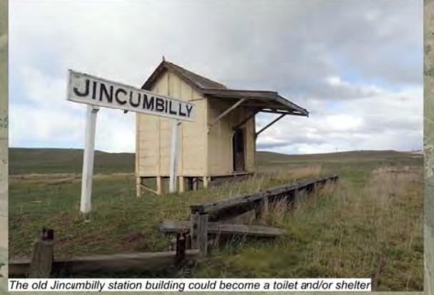
The old Jincumbilly station building could become a toilet and/or shelter
