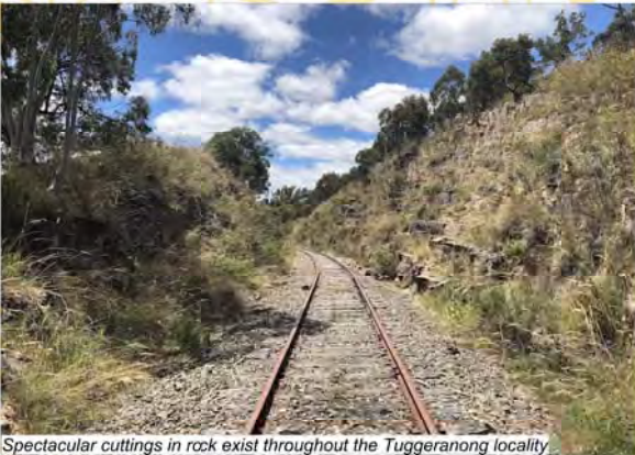
Spectacular cuttings in rock exist throughout the Tuggeranong locality
